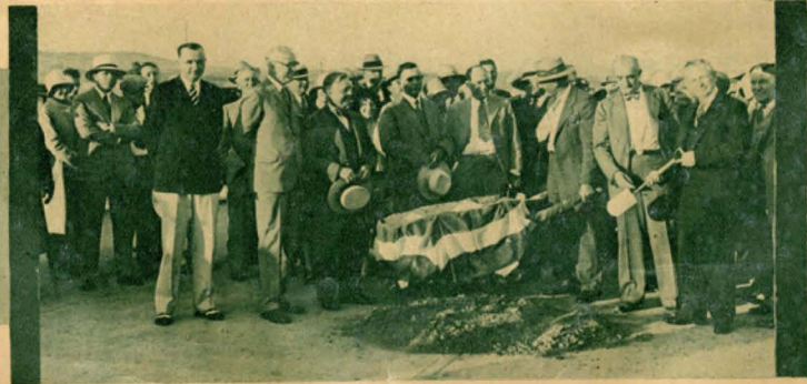
Governor C. C. Young about to remove the last barrier from the paved Roosevelt Coast Highway through Dana Point.
